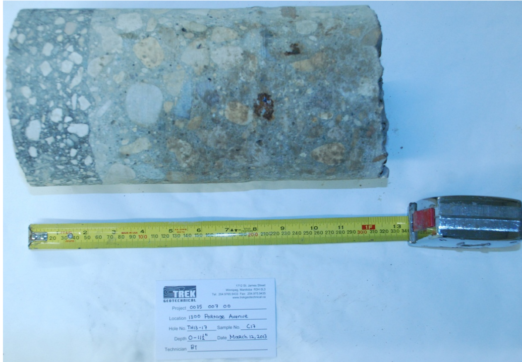
Photo 17: Asphalt and Concrete Core Sample from Test Hole TH13-17
